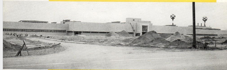
The exterior of the main manufacturing building at the Portage Road Plant is nearing completion and landscaping of the area in front of the building is now under way. The main floor windows at the left end of the building are those of the Printing Department.
