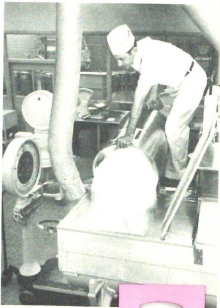
Leo Lemmer portrays early stage in tablet manufacture—blending powdered materials in 600 lb. mixer.
