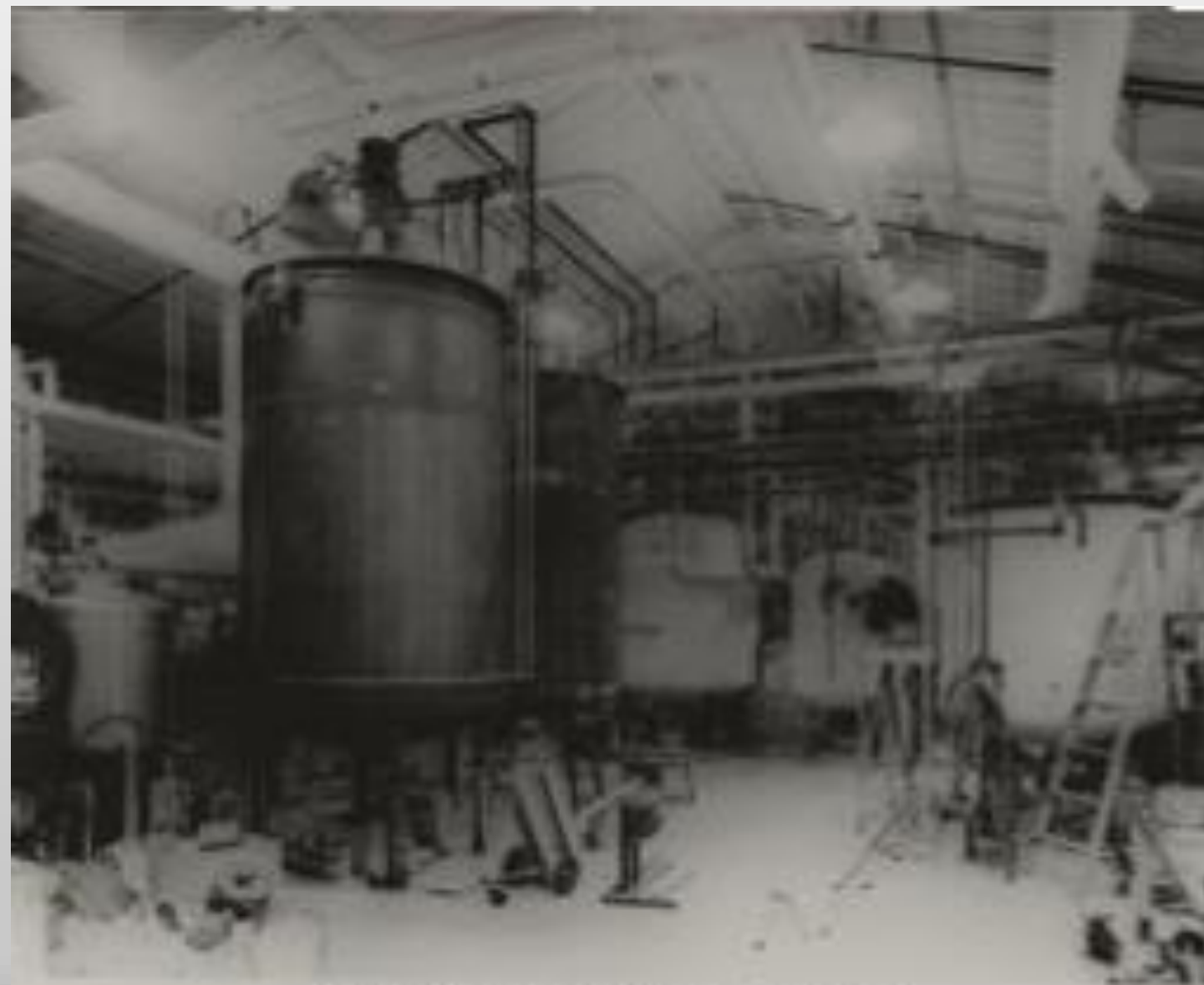
INTERIM CORTISONE PLANT BUILDING 44
